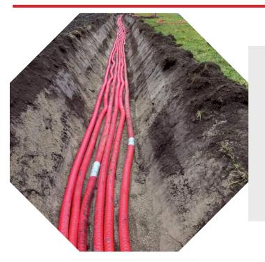
Super Corflo products are extensively utilized in a diverse range of electrical infrastructure projects, including utility work, home construction, telecom, fibre optic Networks, EV charging systems solar farms and retail fueling stations.
